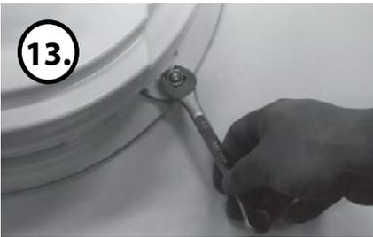
Attach the antenna to the mounting plate
