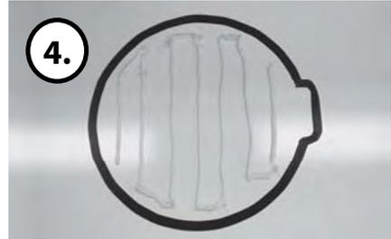
Apply silicone within the guided tape line but leave 2cm gap from the line.
